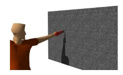
2. Cut along the line making sure the utility knife cuts the material completely.
