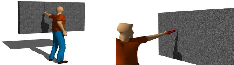
2. Cut along the line using the utility knife. With the thicker foams it may take several passes to completely cut.
